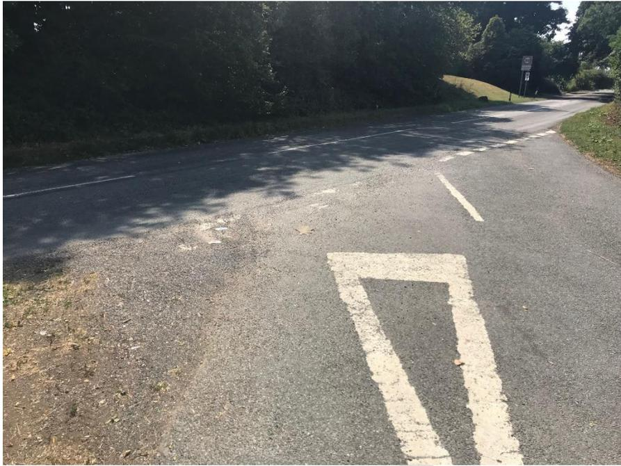
As you can see the angled nature of the junction means that the view from the cab of a horse lorry or similar vehicle would be highly restricted and in essence the similar to that of a left hand drive lorry at a UK roundabout.
